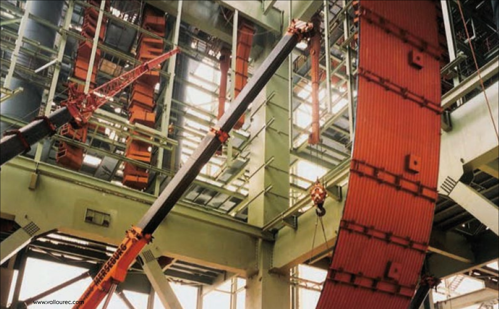
Erection of a water wall in a coal-fired thermal power plant.
