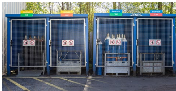
Fig.: Gas storage
