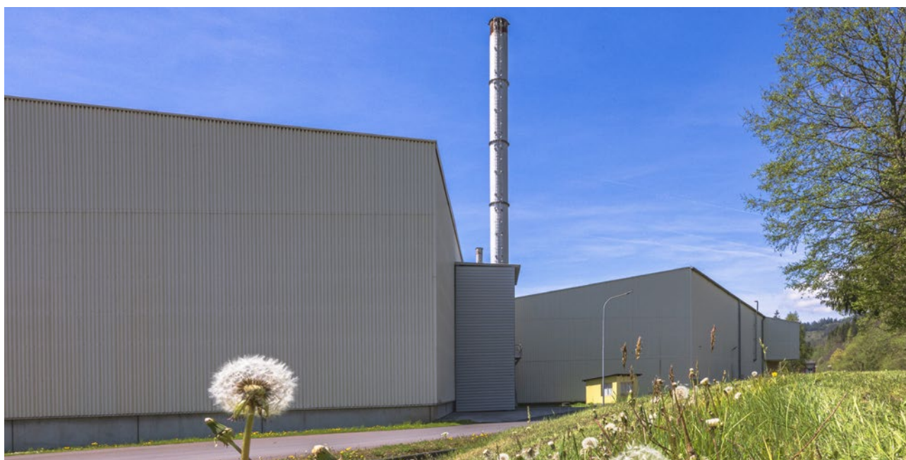
Fig.: Exhaust chimney for heat treatment plant 1
