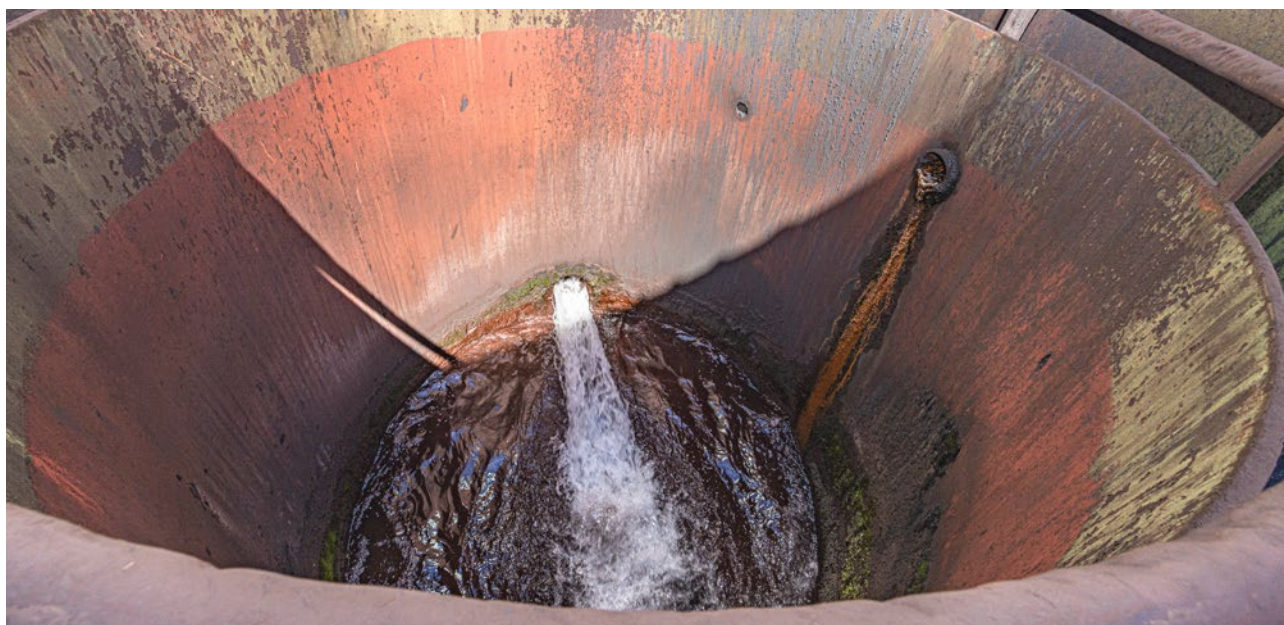
Fig.: Scale trap in CT plant water management system (partial flow 1)
