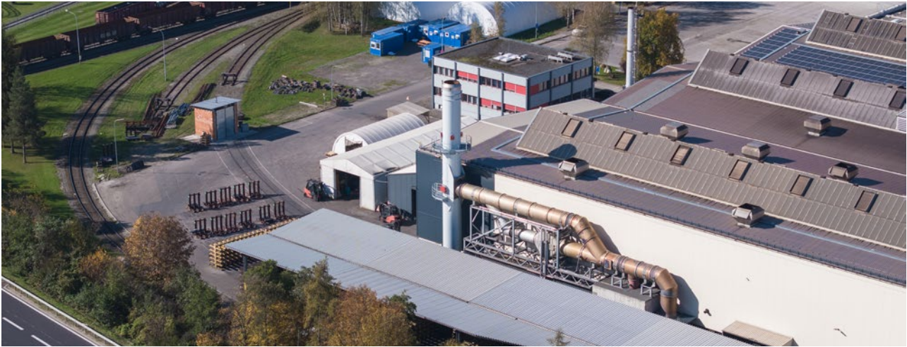
Fig.: Rotary Hearth Furnace exhaust stack with heat recovery
