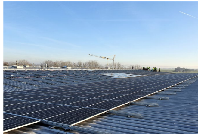
SOLAR PANELS MOUNTED DIRECTLY TO PURLINS
