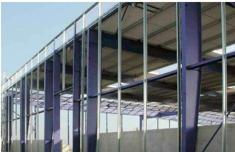
For large industrial buildings it may be advisable to widen the frame spacings to 10 - 18 m, which could then lead to additional columns being required in the long walls.
