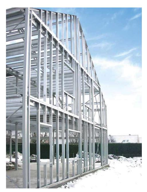
Our wall framing elements are specially developed for external walling and for internal load bearing partition walls.
