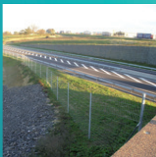
SITES ROUTIERS AUTOROUTES
