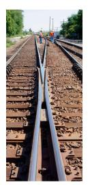
voestalpine Nortrak's Welded Boltless Manganese Frogs (WBM) eliminate all rail joints on the frog providing a continuous running surface unaffected by CWR stresses. This design is used in Class 1, heavy haul service and all passenger rail environments from Streetcar to Commuter Rail due to the smooth transitions and reduced maintenance. This frog design with "flange bearing" properties has been used extensively in embedded applications for LRT and Streetcar.
