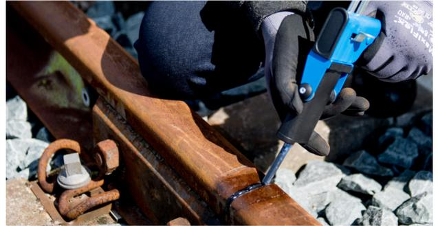
6. Within 30 seconds of filling the joint, place the notch of the scraper in the center of the gap at the bottom of the rail head. Move the scraper over the head of the rail in one movement in the opposite direction as the repair material was applied (eg. from field side towards gauge side). This movement will seal the repair material and form a small bulge which protrudes just above the top of rail. The **Glued Rail Joints Repair** cures within 2 minutes\*.
