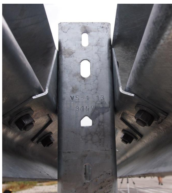
Figure 7: Bolting of intermediate upright
