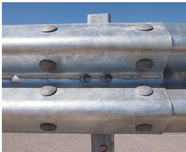
Figure 5: Bolting of jointed area
