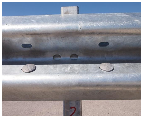
Figure 6: Bolting of intermediate upright
