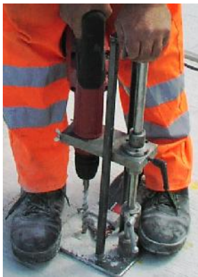
drilling bore hole
