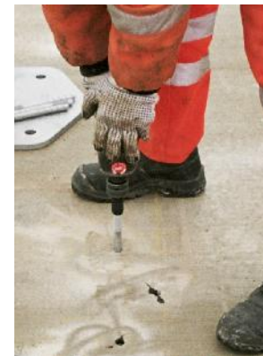
screw the concrete anchor
