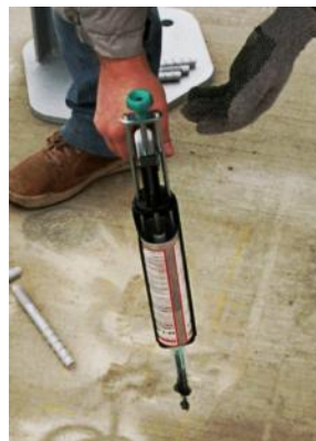
inject the compound mass
