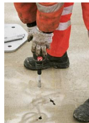
screw the concrete anchor
