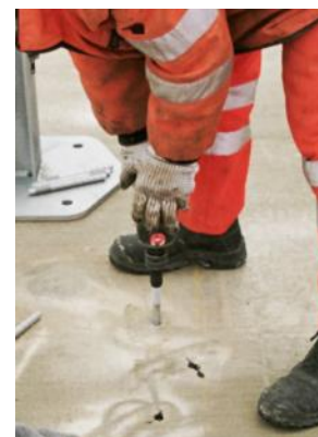
screw the concrete anchor
