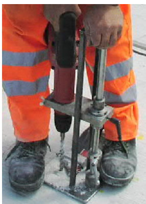
drilling bore hole
