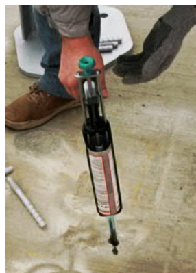
inject the compound mass
