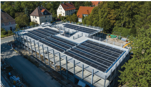
98 kWp, concrete roof GOLDBECK GmbH
