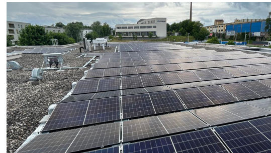
124,67 kWp, gravel roof @ eco-tec.at Photovoltaics GmbH
