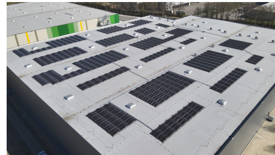
557 kWp, foil roof @ SUNKON GmbH
