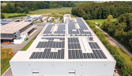
262 kWp, extension, foil roof @ GOLDBECK GmbH
