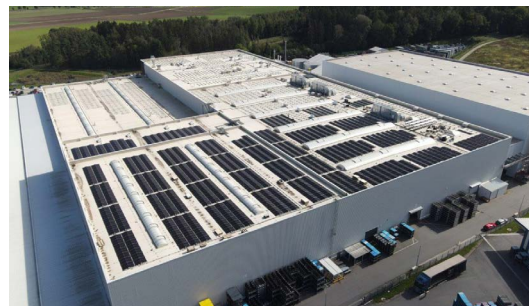
2,0 MWp, tetto in laminato Solarwerk GmbH
