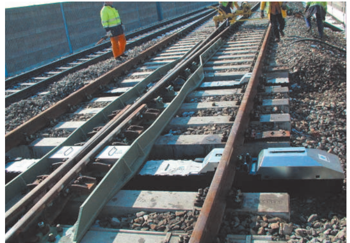
Figure 7: HYDROSTAR® MPF, installed, before tamping
