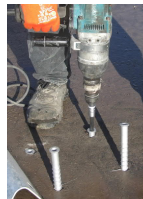
screw the asphalt anchor
