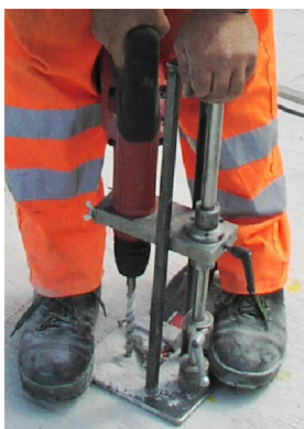
drilling bore hole
