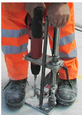
drilling bore hole
