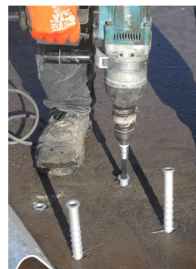
screw the asphalt anchor
