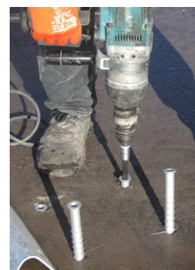
screw the asphalt anchor
