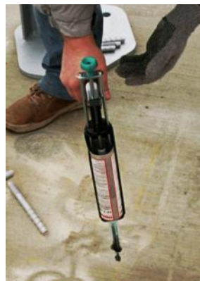
inject the compound mass
