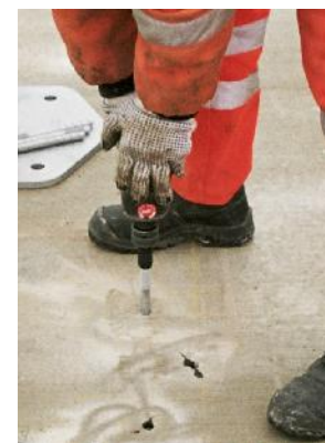
screw the concrete anchor
