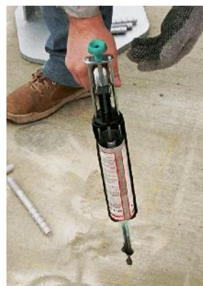
inject the compound mass
