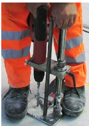
drilling bore hole
