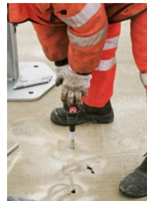
screw the concrete anchor
