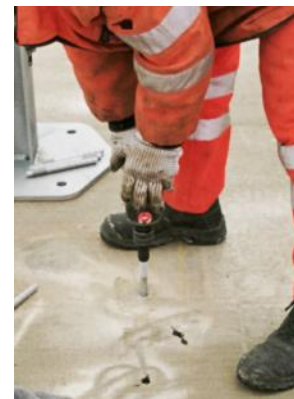
screw the concrete anchor
