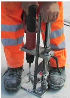
drilling bore hole
