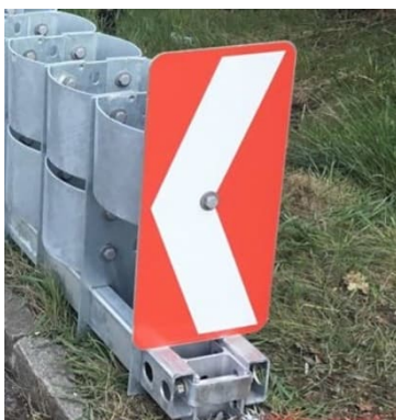
Figure 26: Bolt connection of the directional plate
