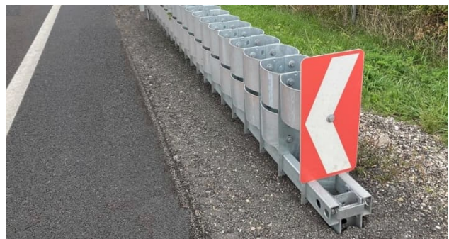
Figure 27: Directional plate alignment
